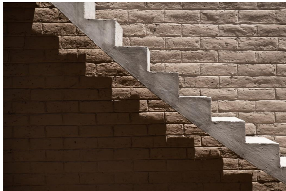
1.32) Escaleras Casa Hilo / Zeller & Moyo Apan, México (ArchDaily / 2019) Arch Daily / https://www.archdaily.mx/mx/923518/casa-hilo-zeller-and-moyo
