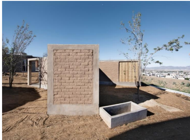
1.31) Vista exterior (patio) / Zeller & Moyo Apan, México (ArchDaily / 2019) ArchDaily https://www.archdaily.mx/mx/923518/casa-hilo-zeller-and-moyo
