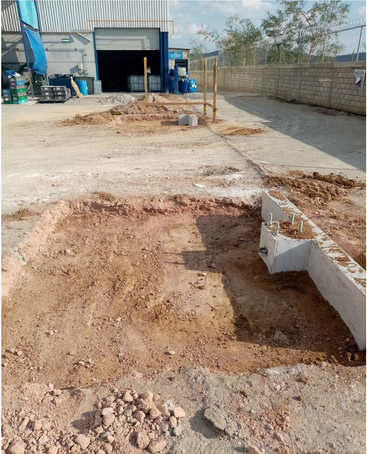
Figura 4.12 Contratraves Nave industrial Amozoc, Puebla
