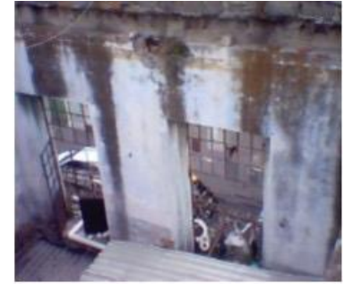
Muro interior de fachada principal
