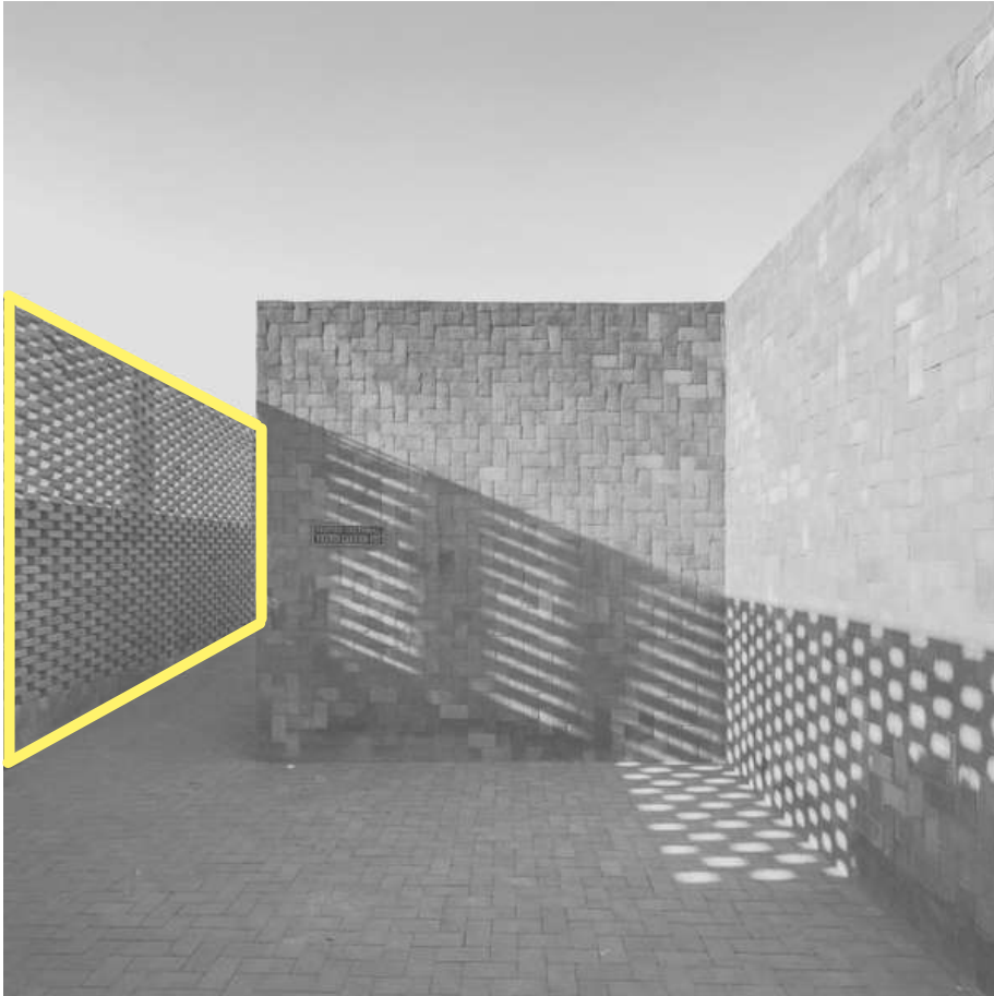
Fotografía: Centro Cultural del Centro Educativo de Morelia, Morelia México. Recuperada de: https://www.archdaily.mx/mx/923997/centro-cultural-del-centro-educativo-de-morelia-ivan-marin-plus-doho-constructivo/5d68a0b1284dd1be600006cb-centro-cultural-del-centro-educativo-de-morelia-ivan-marin-plus-doho-constructivo-foto
