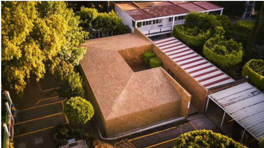
Fotografía: Centro Cultural del Centro Educativo de Morelia. Morelia México. Recuperada de: https://www.archdaily.mx/mx/923997/centro-cultural-del-centro-educativo-de-morelia-ivan-marin-plus-doho-constructivo/5d68a0b1284dd1be600006cb-centro-cultural-del-centro-educativo-de-morelia-ivan-marin-plus-doho-constructivo-foto
