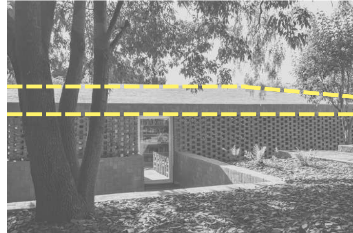
Fotografía: Centro Cultural del Centro Educativo de Morelia. Morelia México. Recuperada de: https://www.archdaily.mx/mx/923997/centro-cultural-del-centro-educativo-de-morelia-ivan-marin-plus-doho-constructivo/5d68a0b1284dd1be600006cb-centro-cultural-del-centro-educativo-de-morelia-ivan-marin-plus-doho-constructivo-foto
