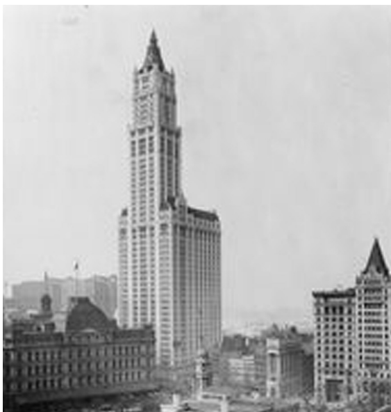
Woolworth Building construido en 1913 en New York, recuperado desde: http://simple.wikipedia.org/wiki/File:View_of_Woolworth_Building_and_surrounding_buildings_New_York_City_1913.jpg
