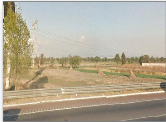
Foto 18: Tramo 14 km 28+200, spor
