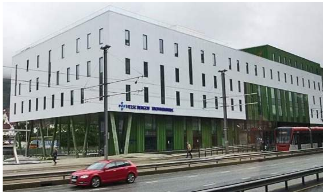
Nota. Adaptado de Kronstadt Psychiatric Hospital, Bergen, Norway . S.f. Manchester History ( https://manchesterhistory.net/architecture/2010/kronstadhospital.html ).
