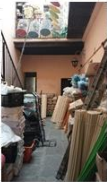
PATIO INTERIOR LAJA SAMBLASTEADA
