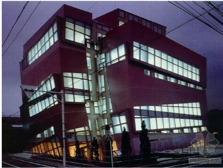
Ilustración 10 Nunotani Headquarters Building
